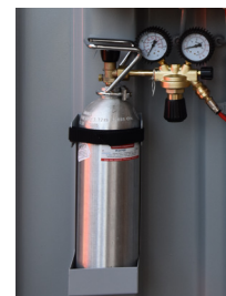
Co 2 pressure cylinder for independent pressure supply
