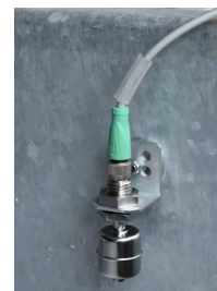
Filling level is mon- itored by probes
