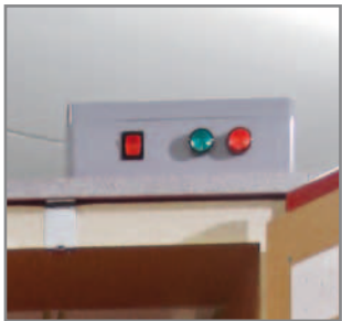
Control unit with fire detection Malfunction message via optical signal and switch-off of the ventilation system.
